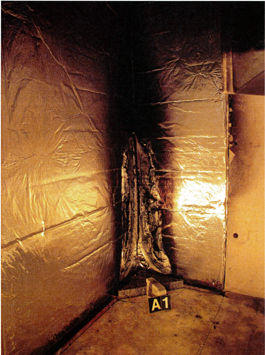
Photo no 3 After test “CR-DUCT”
